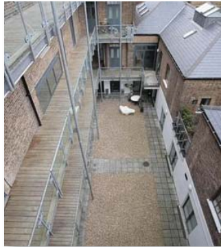
Project: East Smithfield
