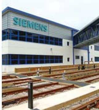
Project: Siemens Northam Depot Southampton
