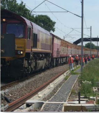
Project: CTRL 105H St Pancras 25KV Diversion Works
